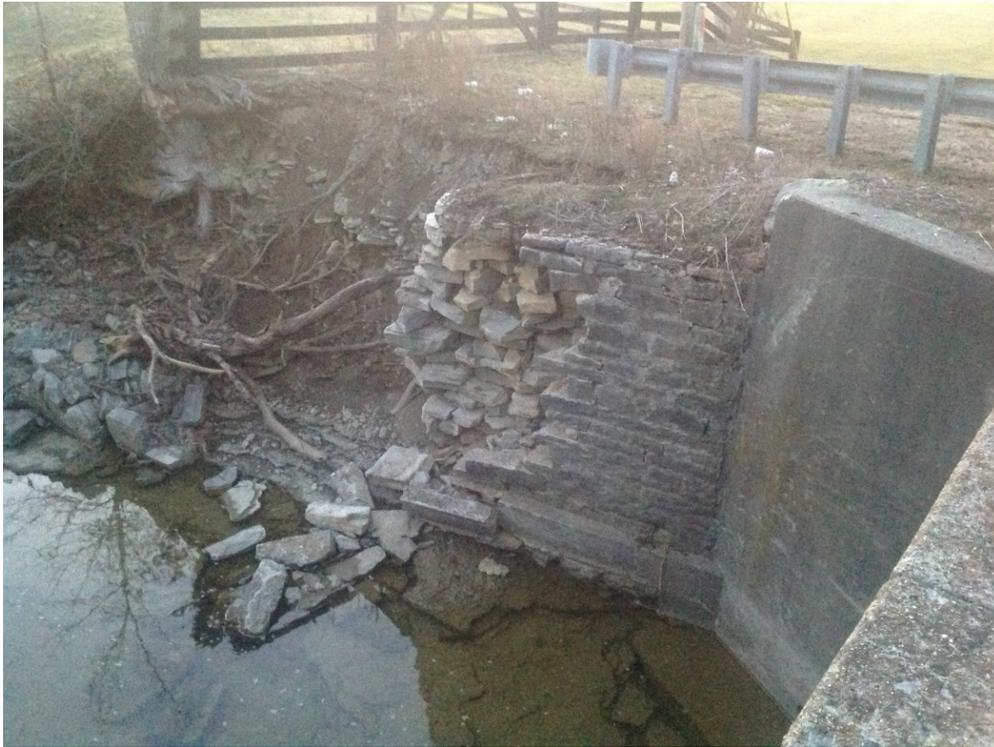
Masonry wing collapsing @ triple barrel culvert near Grundy Home Road
