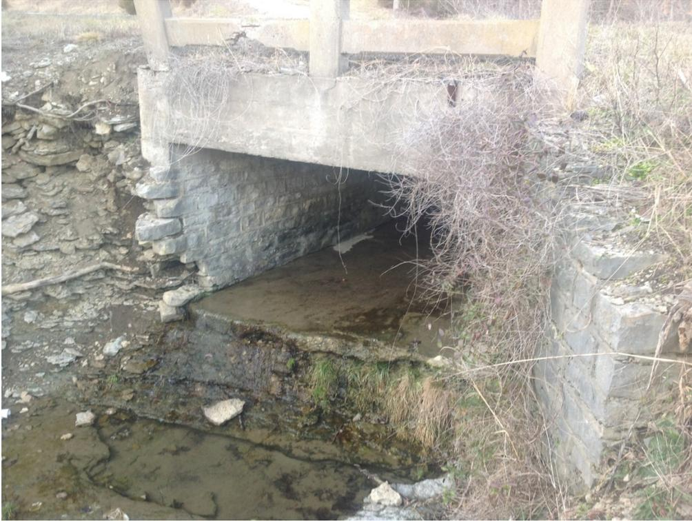
Outlet of existing culvert – rock scour of thin layers and partial collapse of wing. Northwest of Mayfield Lane
