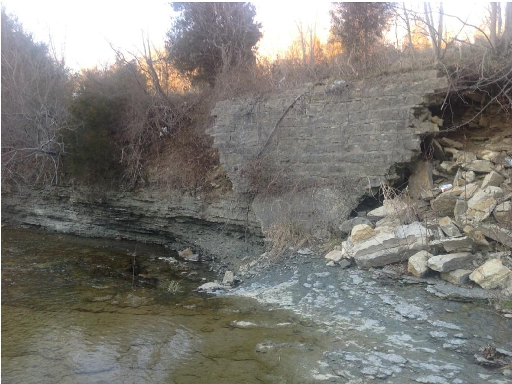
Wall collapsing due to rock scour northwest of Mayfield Lane
