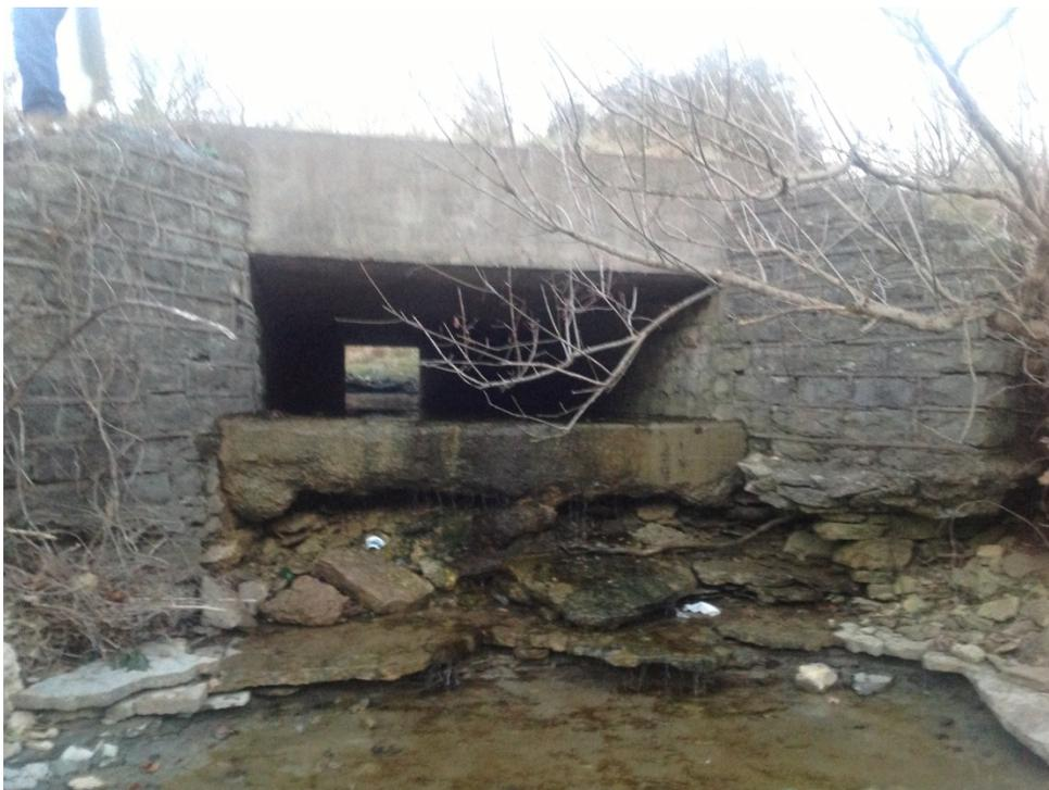
Another Culvert northwest of milepost 3 - slab and wings undermined
