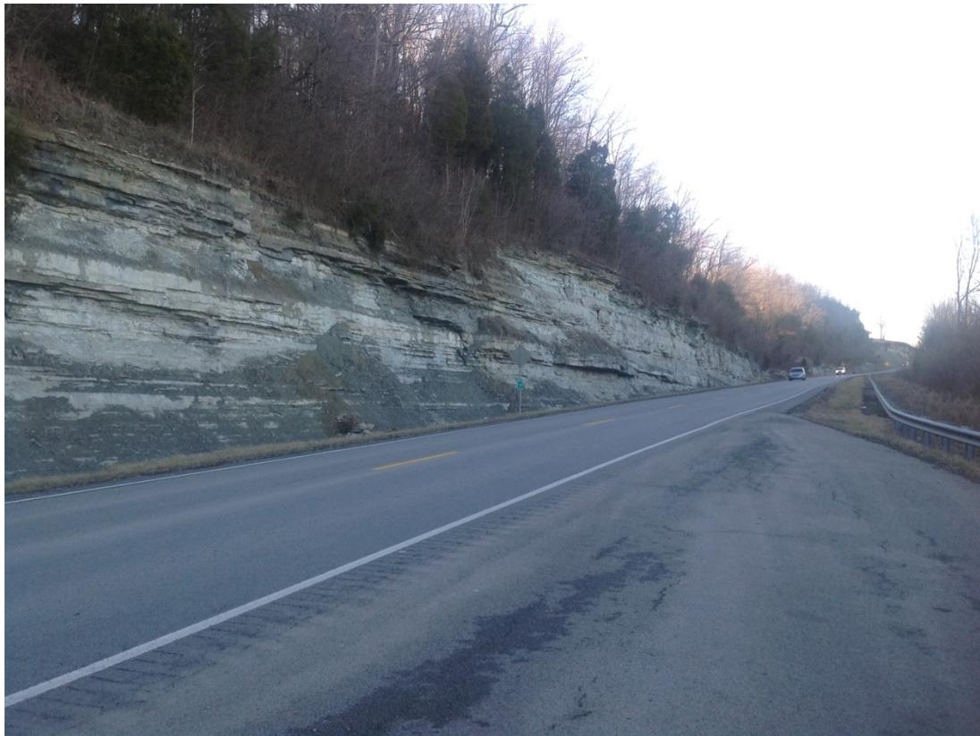
Potentially substandard rock cut (picture near m.p. 7) in the Drakes Formation (Saluda, Bardstown and Rowland Members). There is a fallen rock zone sign near the cuts end.
